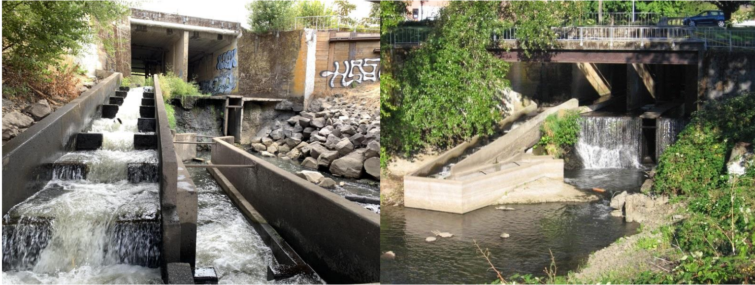
Figure 1. Photographs of the Kellogg Dam fish ladder (left) and view of the complete Kellogg Dam structure just beneath McLoughlin Boulevard in Milwaukie, Oregon.
