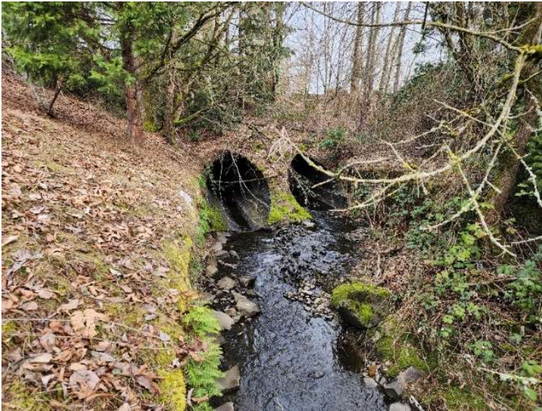
Photo 22. Two CMP's at relatively high slope and no substrate through entire length. Fill at upstream end of culvert to left forces most flows through the culvert on the right.
