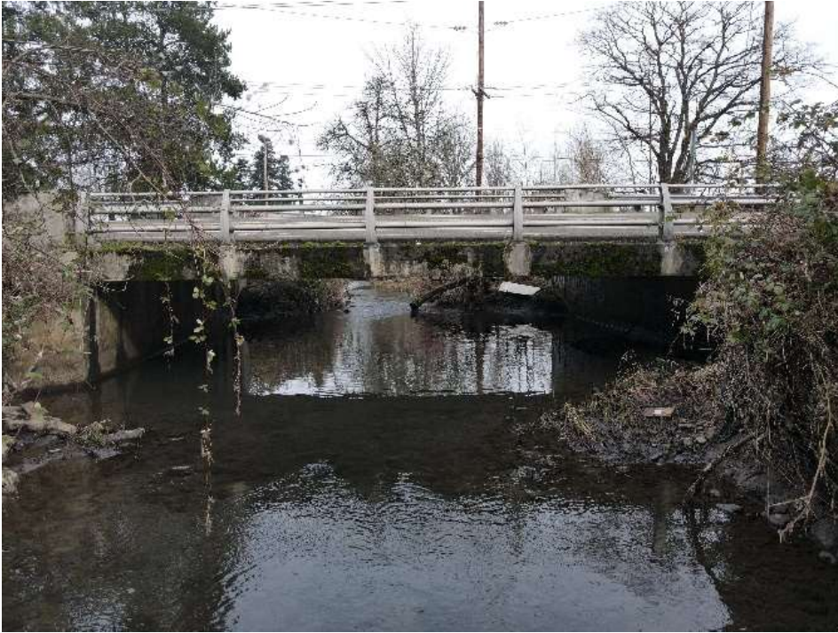
Photo 5. View looking upstream at the SE Lake Road crossing of Mt. Scott Creek. Bridge abutments are within active channel, but they appear to have limited potential to impact upstream migration.
