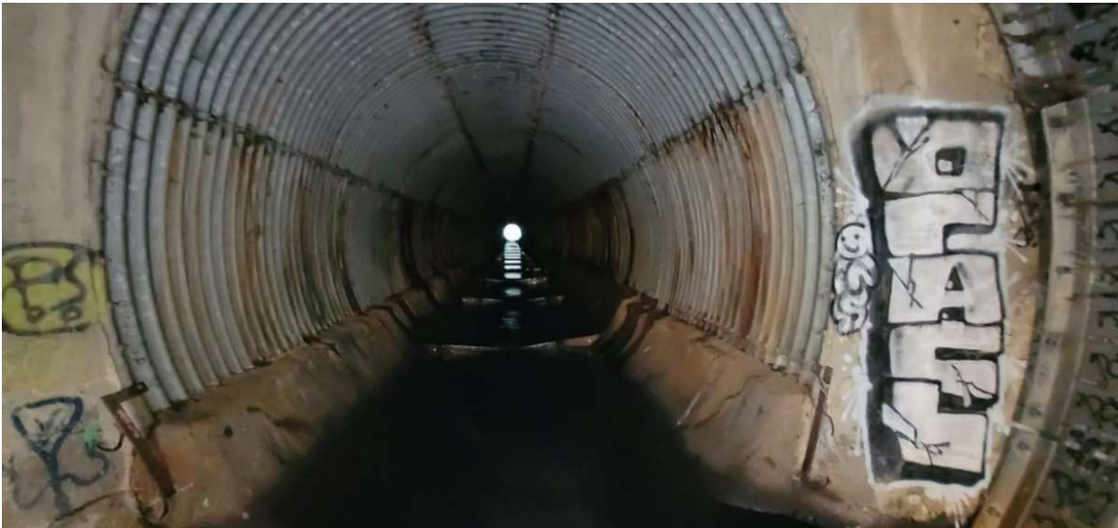
Photo 13. I-205 culvert showing baffles installed to improve upstream passage (upstream view)
