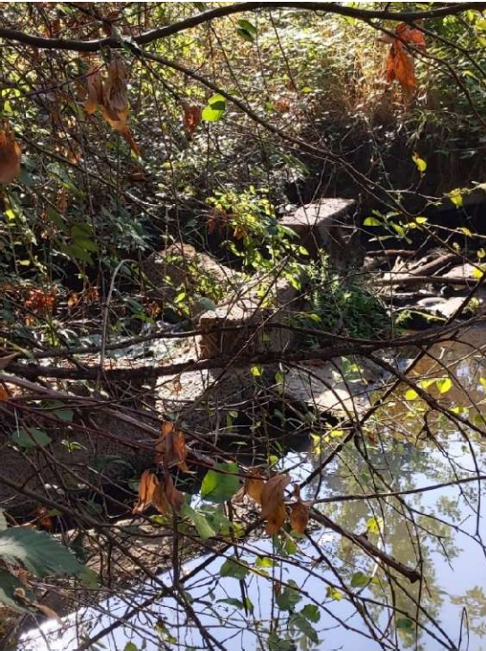
Photo 7. Water control structure. Notice damage to structure at far bank. The left bank is eroding at an unnatural rate because of the failing structure. It is not clear the purpose of the structure or who built it.
