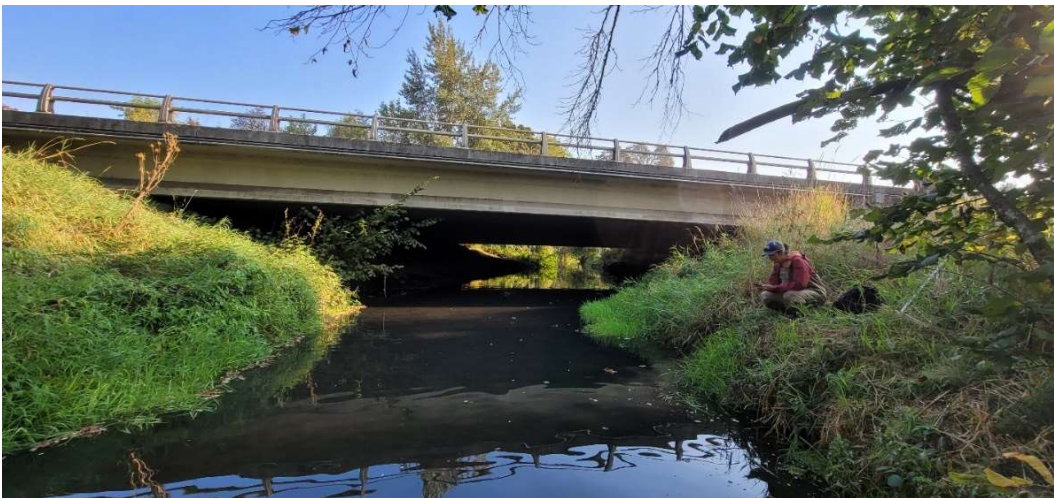
Photo 3. Upstream view of the Highway 224 crossing of Mt. Scott Creek. Bridge fully spans natural stream channel below.
